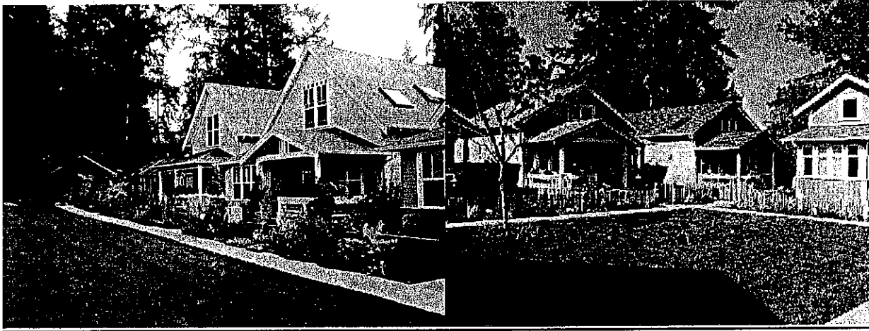
Figure 2. Cottage development examples. Note common open spaces and porches and semi-private open spaces oriented towards the commons.
