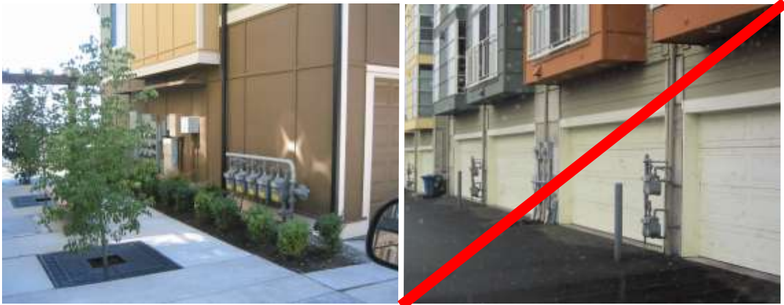
Figure 33. Good and bad utility meter configurations. The examples on the left are consolidated and somewhat screened by landscaping elements, whereas the right examples are exposed and degrade the character of these townhomes.
