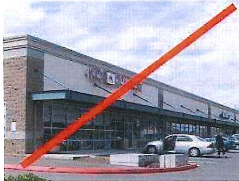
Figure 39. Facades that meet (top image) and don't meet (bottom image) the storefront articulation standards. The top image uses repeating window/storefront patterns, separate weather protection elements, and vertical piers to successfully articulate the facade. The bottom image uses continuous window and weather protection elements and thus wouldn't comply with the standards.
