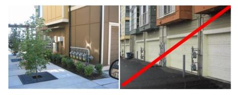
Figure 33. Good and bad utility meter configurations. The examples on the top are consolidated and somewhat screened by landscaping elements, whereas the bottom examples are exposed and degrade the character of these townhomes.
