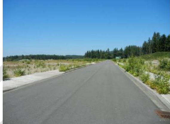
View of developed road and sidewalk infrastructure
